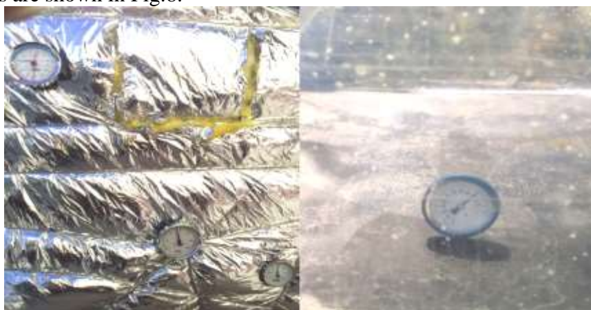
Fig.8. Temperature field in a laboratory installation
